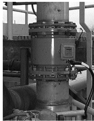
Left: Flow tube replaces inefficient control valve. Above: PumpSmart intelligent flow control system will save $30,000/yr.
